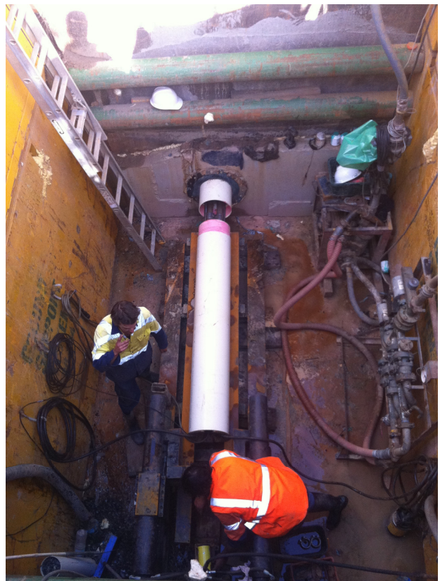
Figures 1 & 2: Images of PVC Jacking Pipe (Photos courtesy of GM Microtunnelling)
