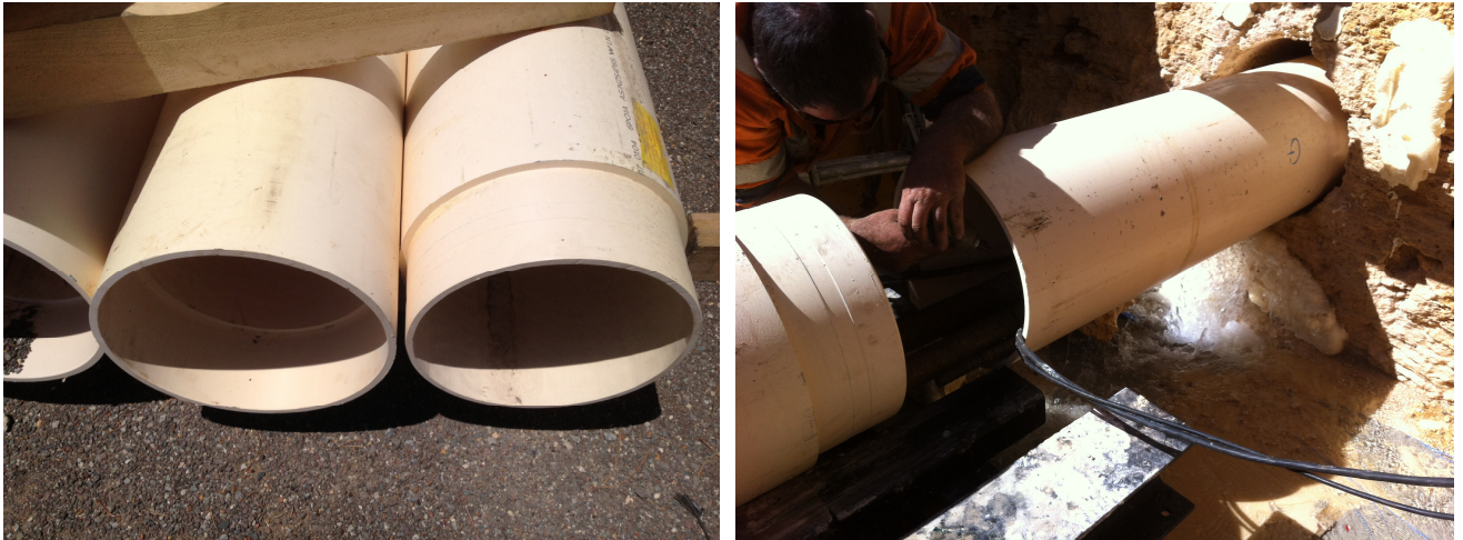
Figures 3 & 4: Ends of PVC Jacking Pipe (Photos courtesy of GM Microtunnelling)
