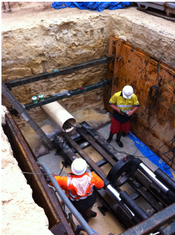
Figures 1 & 2: Images of PVC Jacking Pipe (Photos courtesy of GM Microtunnelling)
