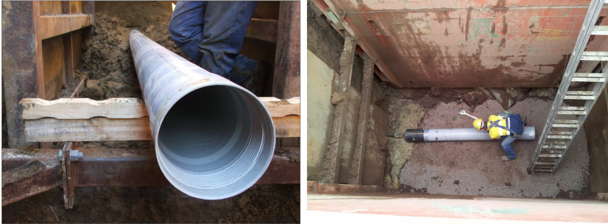
Figures 8 & 9: Segmental Sliplining pipe (Photos courtesy of Iplex Pipelines)
